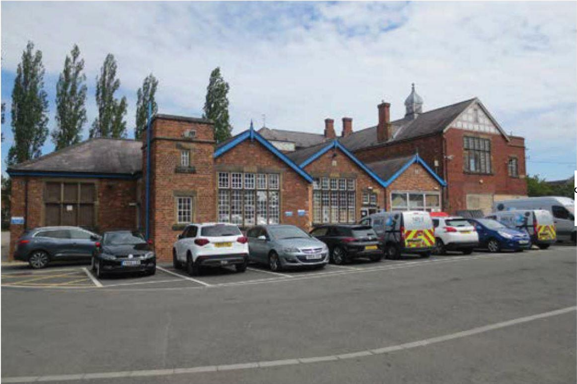
Existing Building - Rear
